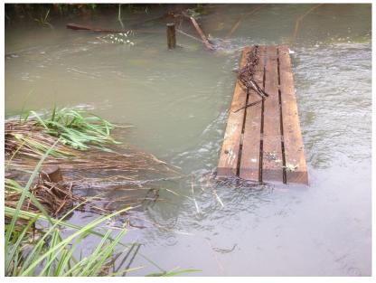
Hamilton City storm water system. This means during heavy rain the water level rises quickly, but equally, as soon as the rain stops the water level quickly recedes. This, and the fact that Hamilton City Council do not approve of fixed structures across their storm water network, led us to design our bridges that would survive these conditions. We are building our bridges out of H3 70 x 100. We put
